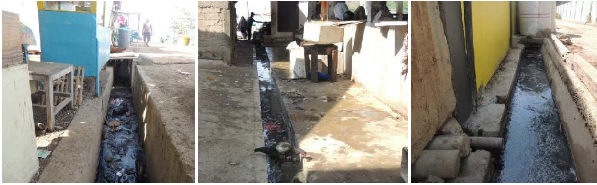
Figure 66: Road ditches in Labuan Bajo's city centre (picture by courtesy of the department of environment)
